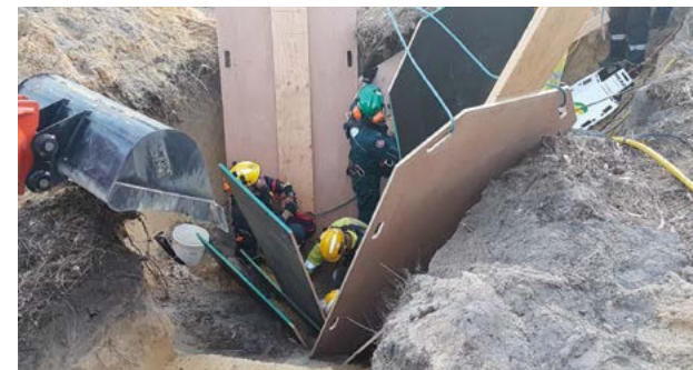
USAR officers providing protection against more sand slippage
