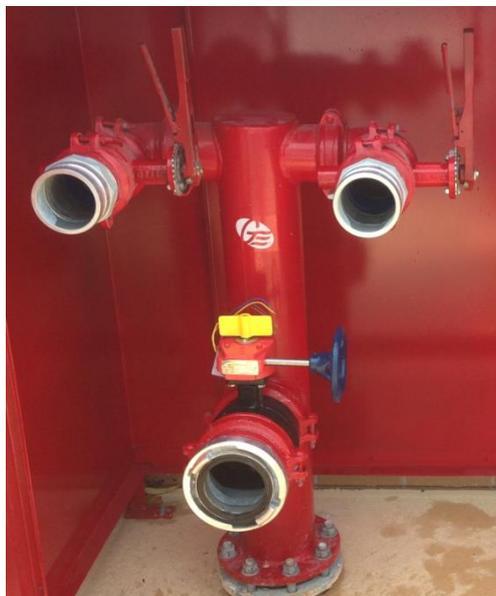
Figure 1.2. Typical 125mm Storz coupling with 100mm male Camlock coupling
