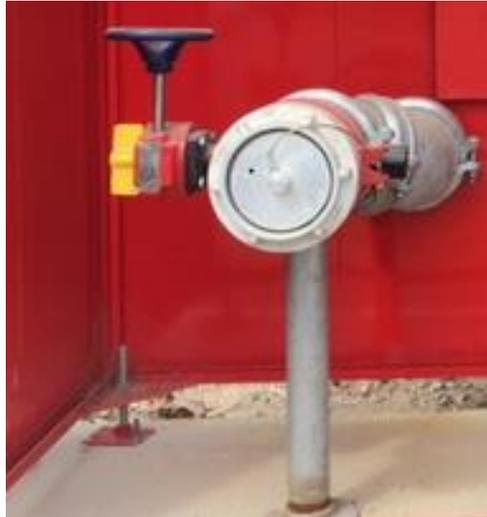
Figure 1.1. Typical 125mm Storz coupling
