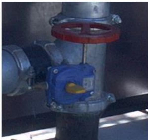
Figure 1.6 Typical isolation valve for a storz connection meeting AS2419.1:2005 requirements.
