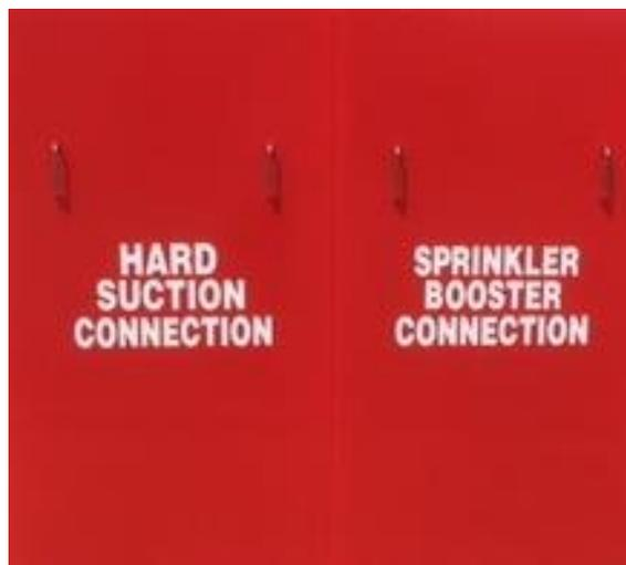
Figure 1.10b. Typical signage to a booster assembly containing a hard suction
