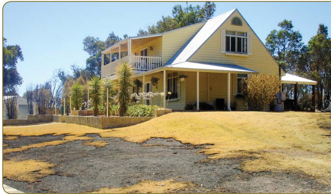
Above: Well prepared Building Protection Zone with reduced fuel.
