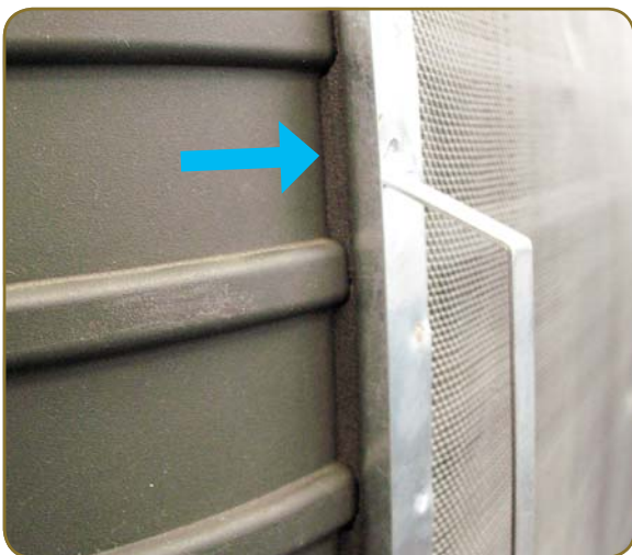
Figure 6. A sealant is used to fill any gaps.
